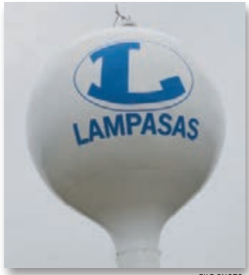
FILE PHOTO An engineering analysis will recommend potential improvements to the water distribution system for western parts of town, which are served by this water tower at Nix Road and North Willis Street.
